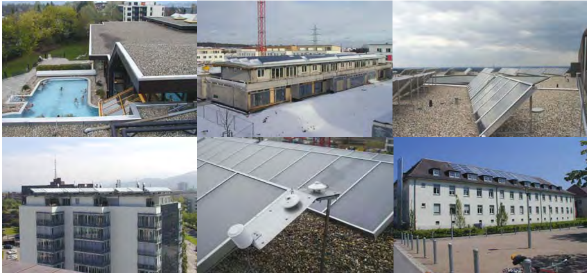
Fig. 1: Photo gallery of the solar systems monitored by Hochschule Offenburg.
