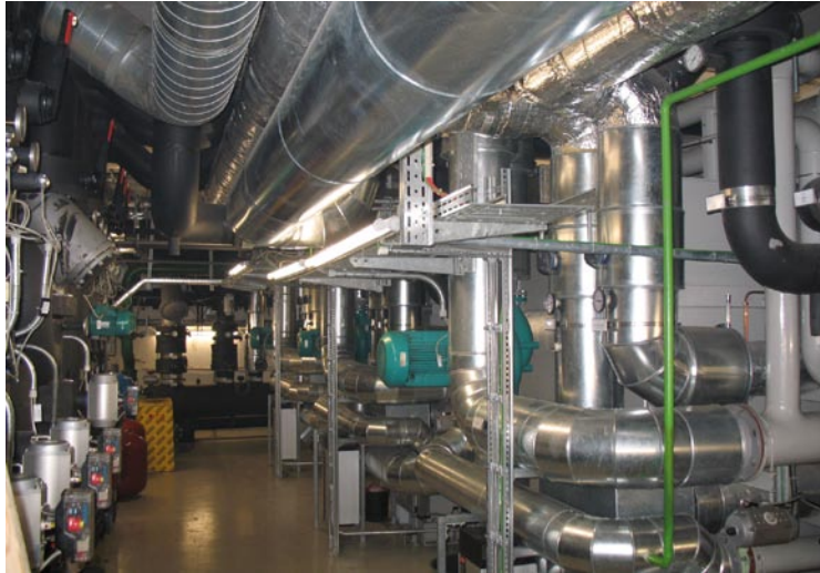
Figure 3: View to the piping of the adsorption chiller at Fest AG & Co. KG.
