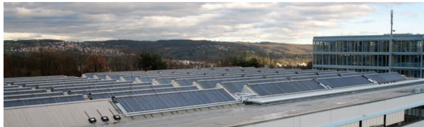
Figure 2: Collector array (1330 m 2 ) at Festo AG & Co. KG
